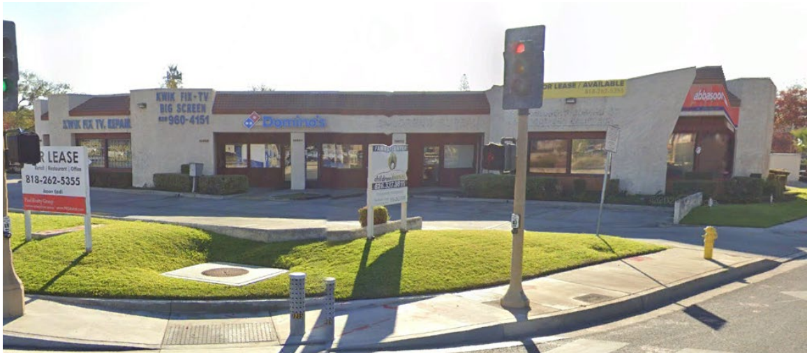
Opportunity Site - 14598 Ramona Blvd, Existing Conditions
